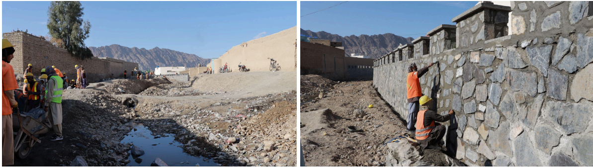
Construction of Teri Ada Protection Wall with total length 350m G5 District #9 Kandahar province on 18 February 2025
