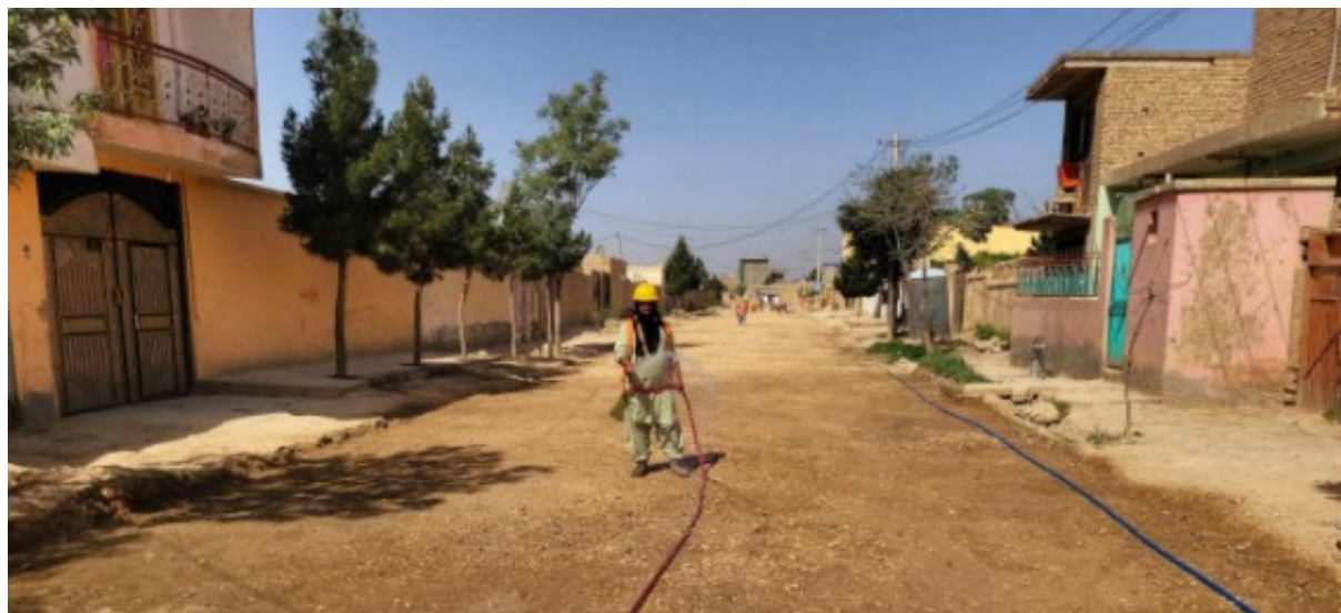
Dust control at the subproject sites.
