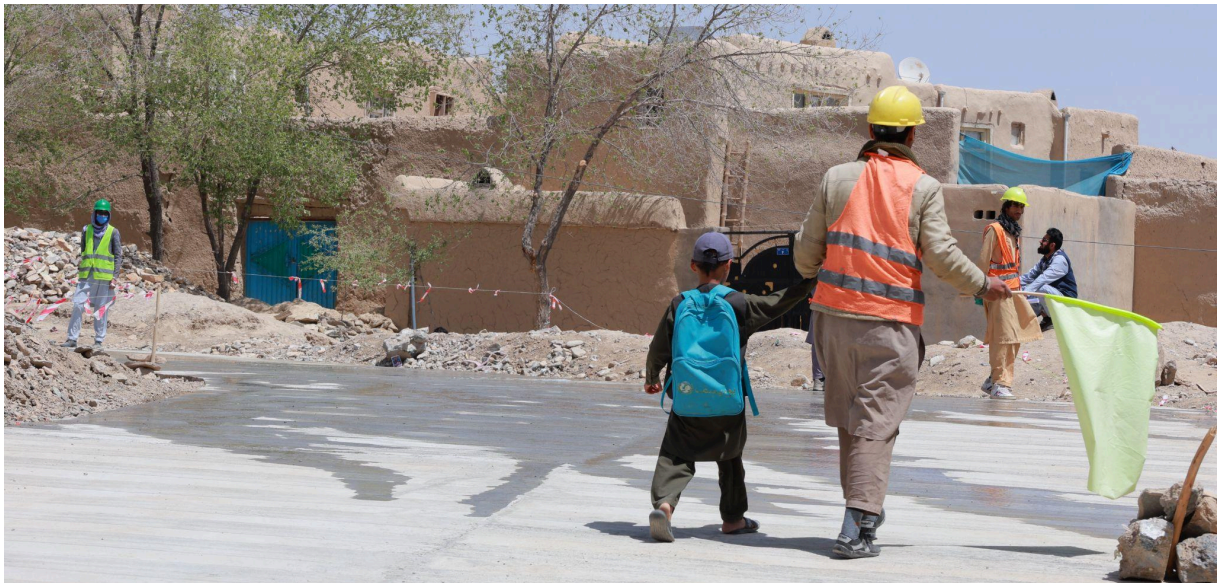
A traffic controller assists a school child to bypass active works at the Construction of Sultan Mahmood plum concrete surface street (L=600m), Gozar #6, District #2, Ghazni city, on 16 April 2025
