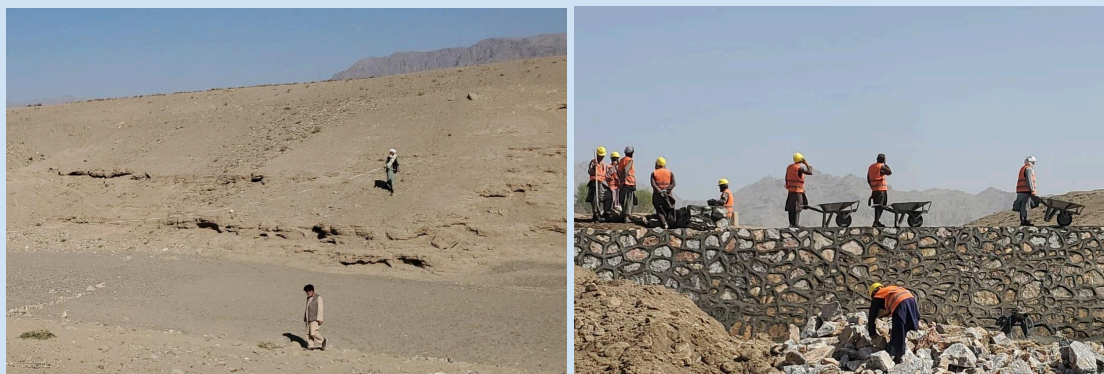
Before project implementation (left) and work in progress (right) at Pir Zada CRG check dam, Maiwand District, Kandahar Province
