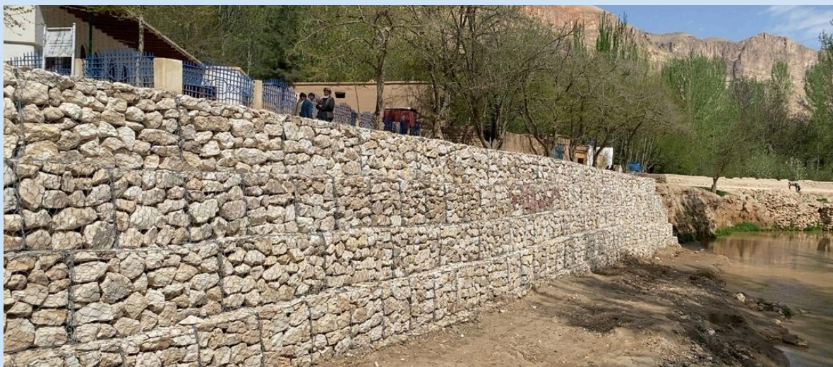
Completed gabion wall
