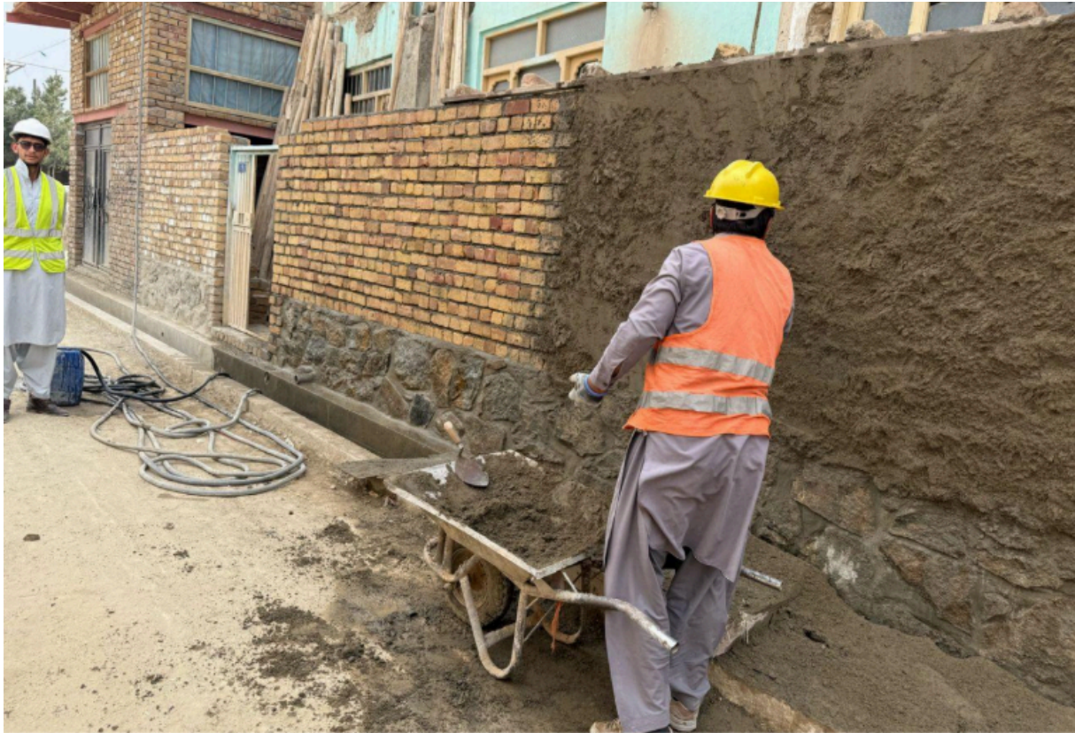
Construction of the boundary at the Sangkashan Project in District 1 of Kabul City, 21 April 2025.
