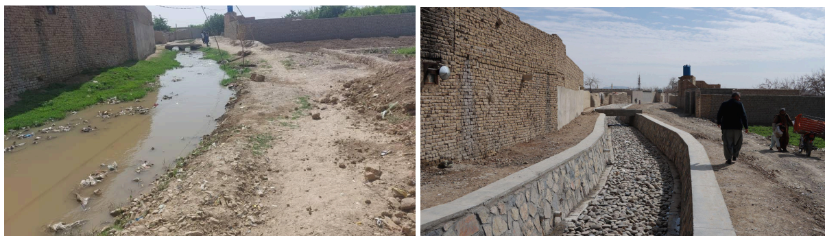
Construction of Mirza Khan Qalacha Drainage Protection Wall With 850m Length in District 13 of Kandahar province on 18 February 2025
