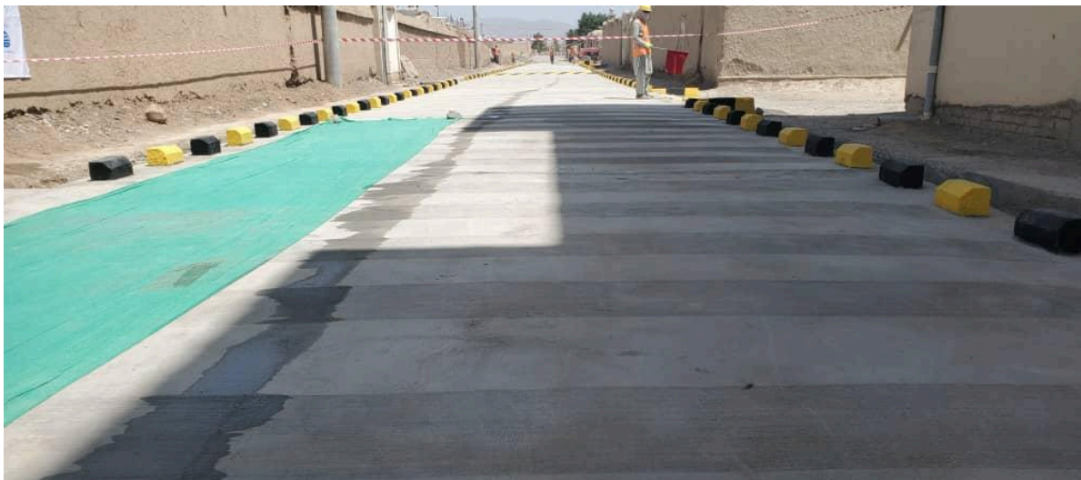
Recently paved street in project Upgrading Street (Part A and B) of Peerbagh with Plum Concrete surface with a total length 556m and additional 20-meter stone masonry wall, Gozar #01, District #03, Gardez City 29 April 2025
