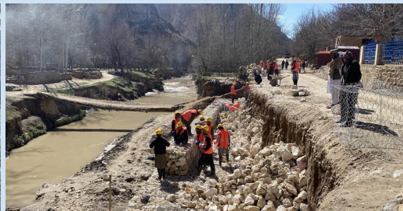
Before implementation of the project in Samangan province (left) Laborers installing the gabion wall (right)
