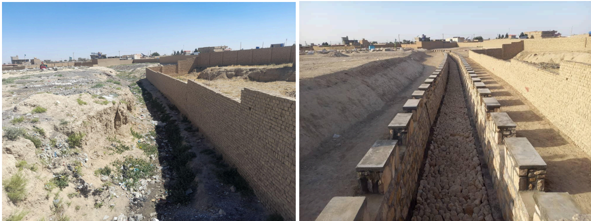
Construction of Abu Talib Guzar Protection wall for flood Control Canal with total length of 300 m, Gozar#11, District#05, Mazar-e-Sharif City
